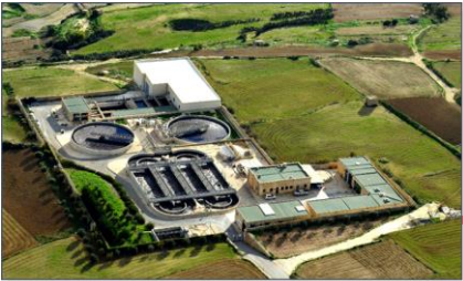
Ras il-Hobz STP (2007) NEW Water Plant (2018) 3200 m3/day
